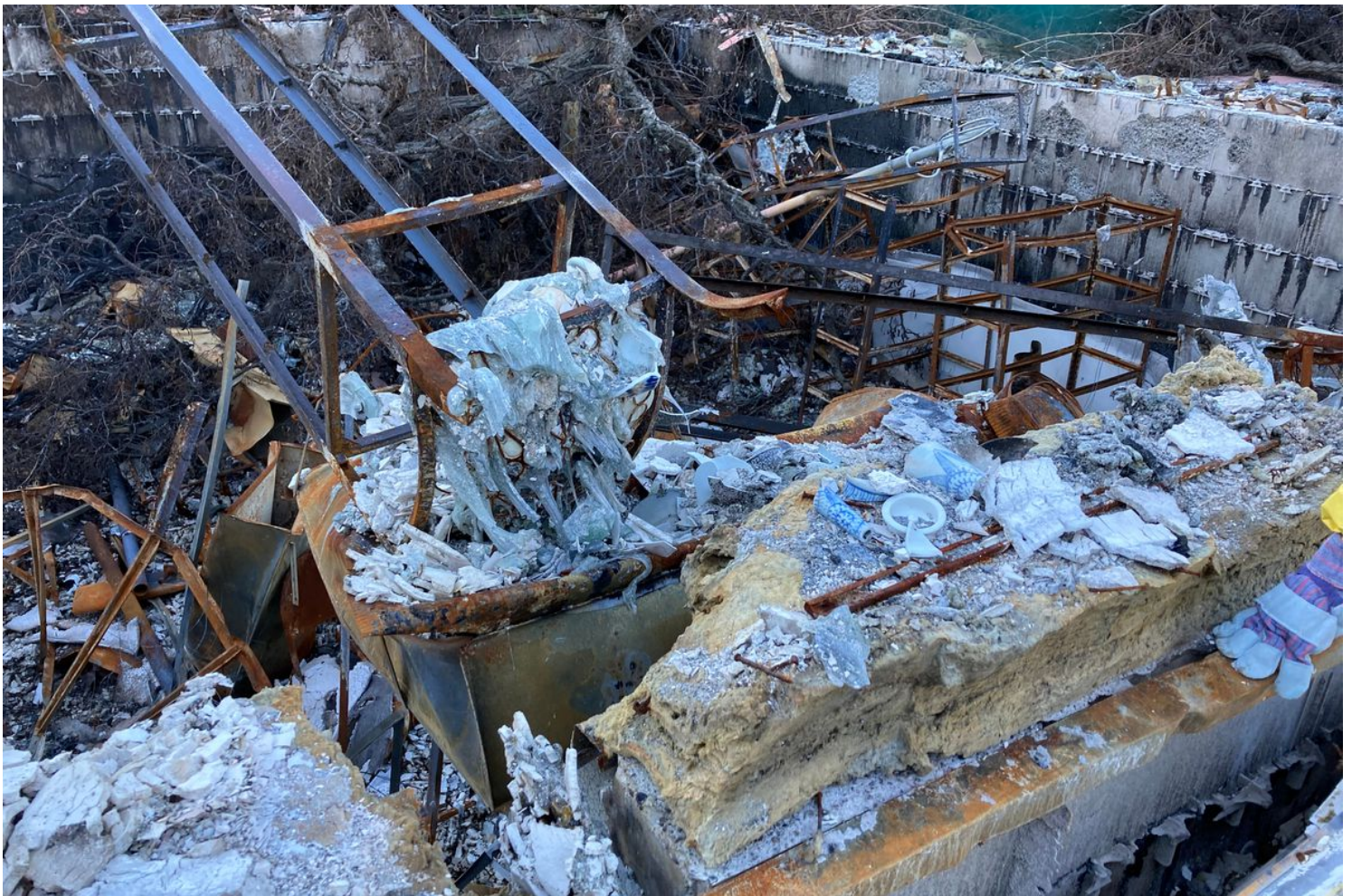
Melted glass and charred metal are all that remains of the Lytton Chinese History Museum.
